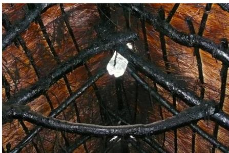
One part of the required material exists in the village (2,5l PET bottle, a piece of old metal) while the rest is cheap and sufficient for several families (chloral and silicon). The lamp was installed on the roof and it had an immediate positive effect as it became significantly lighter. The family was really enthusiastic and especially Margarita who said that now she could really see something while cooking!
